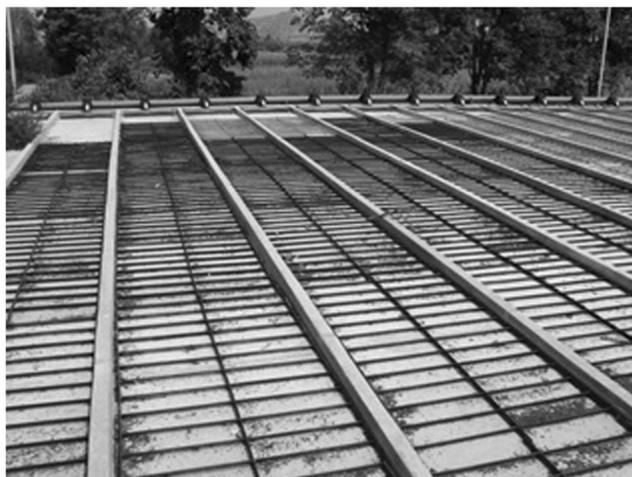
**Fig. 4** The large-scale cultivation plant with a total area of 3000 m<sup>2</sup> made of concrete was constructed in Rupite, southwest Bulgaria. It consisted of thin-layer sloped platforms placed on the ground over which microalgae would flow. The platforms had a slope of 3% and were fitted with transversal baffles to increase culture turbulence
