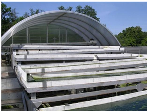
**Fig. 11** A multiple-lane cascade system constructed as a semi-closed system placed in a greenhouse (Institute of Microbiology, Třeboň, Czech Republic). The culture was circulated over the cascade of 8 smooth polypropylene platforms arranged in a meandering way with a declination of 1.6% (total area of 56 m<sup>2</sup> and total volume of 500–600 L) which were connected by troughs. The flow velocity was about 0.5 m/s with a culture layer thickness of about 6–7 mm
