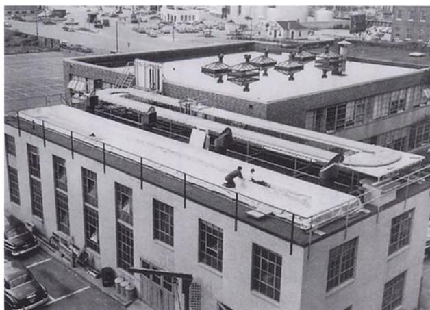
**Fig. 1** One of the first pilot-scale units (about 4000 L) was devised and tested at Arthur D. Little, Inc. in Cambridge, Massachusetts in collaboration with the Carnegie Institution in 1951. The photobioreactor was formed by a loop of thin-walled polyethylene tube of a 7–8-cm depth with continuous circulation of the culture by a pump
