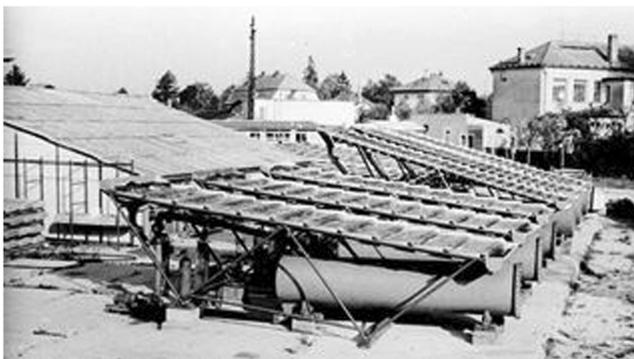
**Fig. 2** First generation of outdoor cascades built in Třeboň in early 1960s
